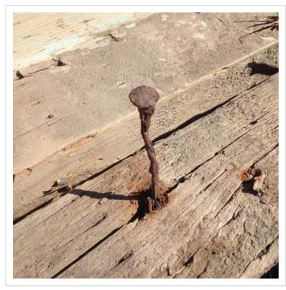
Corroded spike for deck board fastening.
