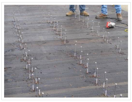
This picture shows the deck fastening in progress. The screws are set and ready for driving with screw-driving tools.
