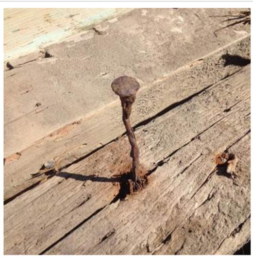
Corroded spike for deck board fastening.
